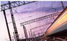
Network Rail | Digital Railway Programme, and Trans Pennine Route Upgrade
